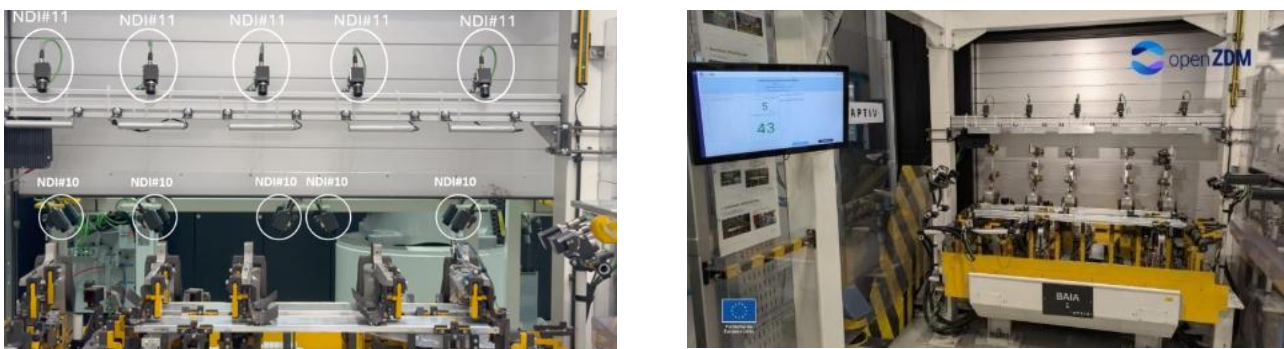
Figure 12: NDI#10 and #11 installed in-line in APTIV (M42).
